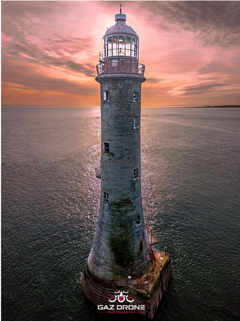
Image of the day – Haulbowline Lighthouse
